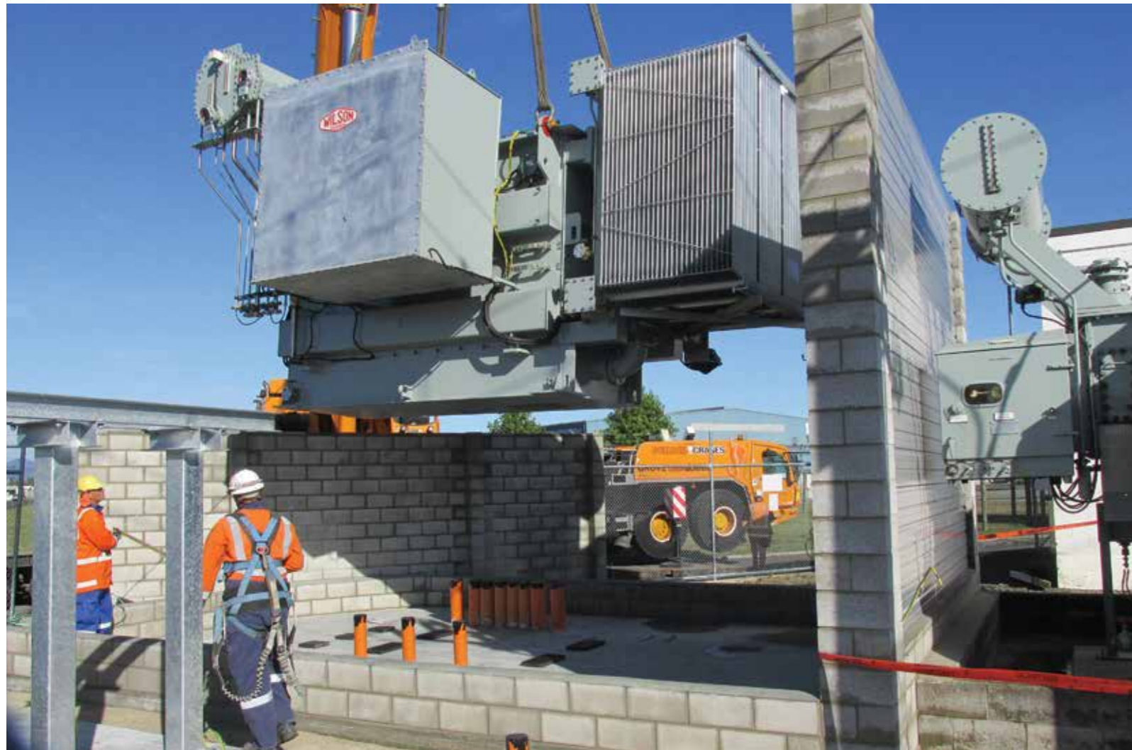
Left: A 17MVA transformer, capable of powering 8,500 households and supporting industrial growth, is lowered into place in Waharoa.
