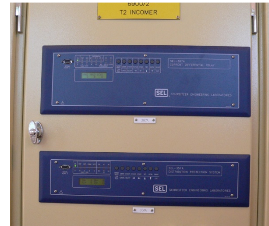
Figure 21.4: Modern numerical relays
