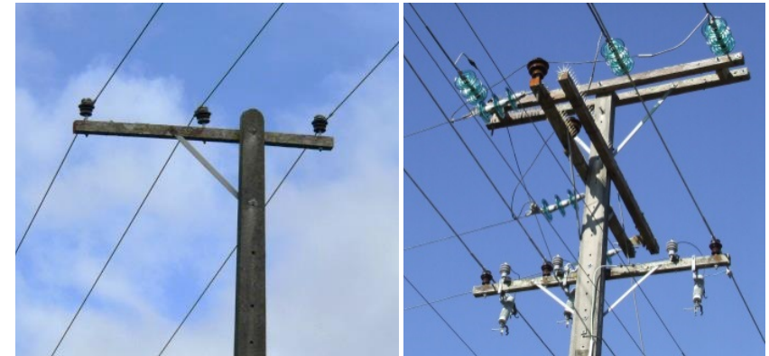
Figure 15.7: Different crossarm configurations
