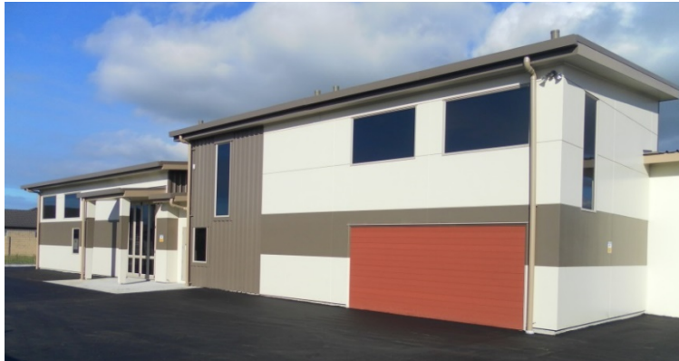
Figure 18.15: Urban zone substation building
