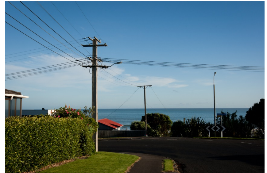
Figure 16.14: LV overhead circuit
