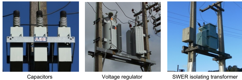
Figure 19.10: Collection of other distribution transformers
