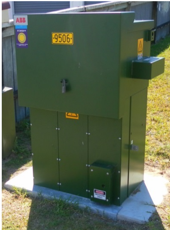
Figure 20.1: Ground-mounted switchgear
