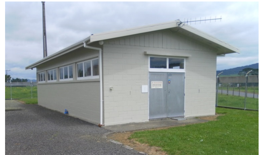
Figure 18.14: Masonry constructed building
