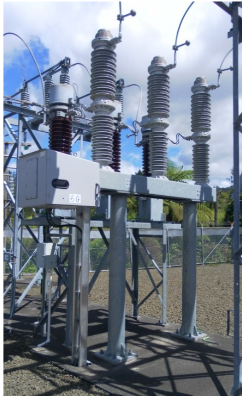
Figure 18.12: Live tank SF 6 outdoor 33kV circuit breaker
