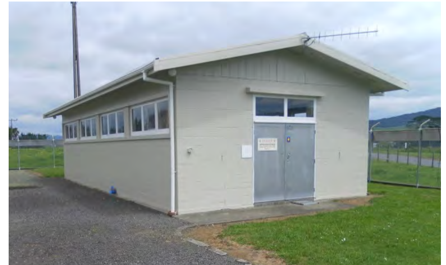
Figure 21.12: Masonry constructed building
