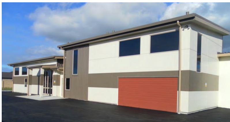
Figure 21.13: Urban zone substation building
