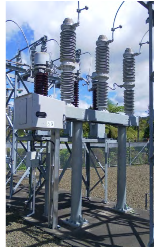
Figure 21.11: Live tank SF 6 outdoor 33kV circuit breaker
