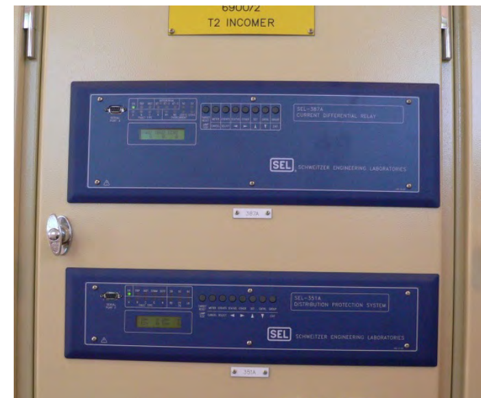
Figure 24.4: Modern numerical relays
