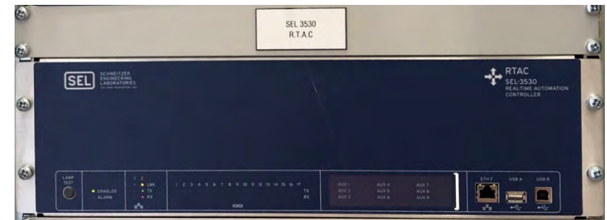
Figure 24.1: A modern RTU
