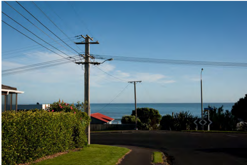
Figure 19.7: LV overhead circuit
