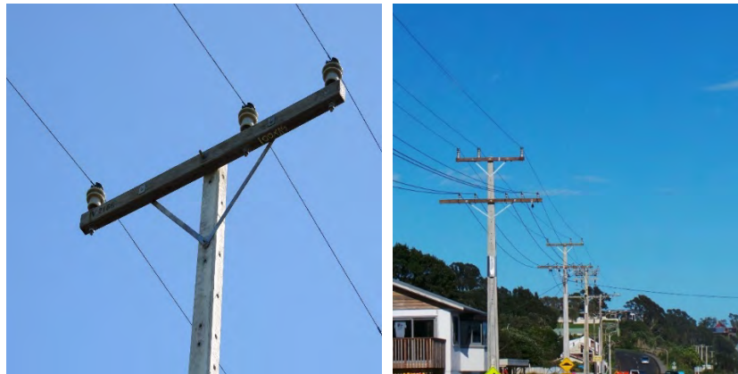
Figure 18.6: Different crossarm configurations
